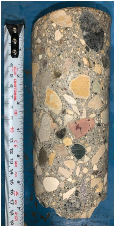
Figure 17 – Core No. 56 (Hood Ave)
