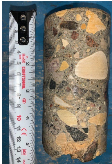
Figure 23 – Core No. 62 (Summerfield Way)
