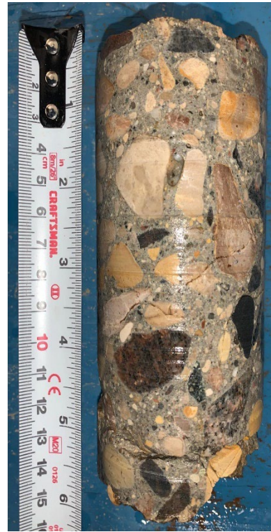
Figure 14 – Core No. 53 (Dahlia Alley)
