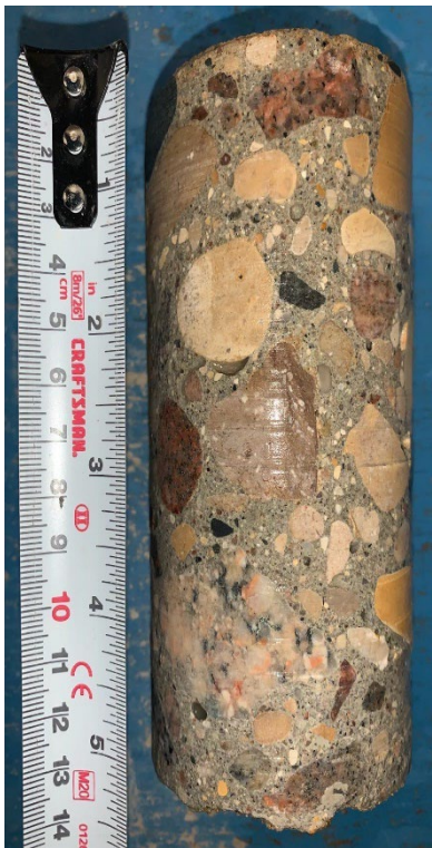
Figure 25 – Core No. 64 (Summerfield Way)
