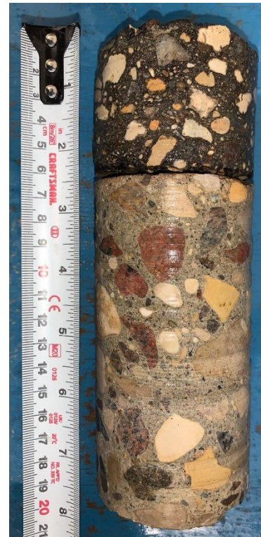
Figure 20 – Core No. 59 (Summerfield Way)
