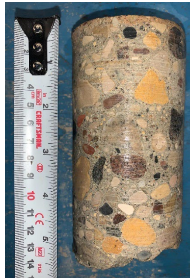
Figure 24 – Core No. 63 (Summerfield Way)
